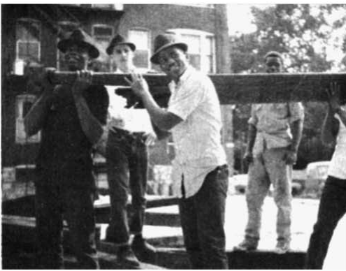
A Neighborhood Commons is lugging railroad ties.
