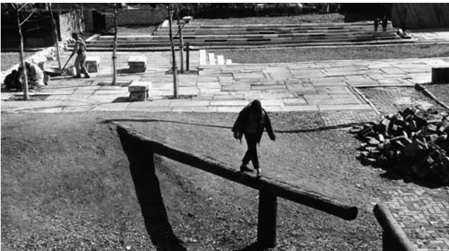
Figure 6 Rescuing salvage, in this case marble steps, for Melon Commons, 1960 (Karl Linn Collection, Environmental Design Archives, University of California, Berkeley).
