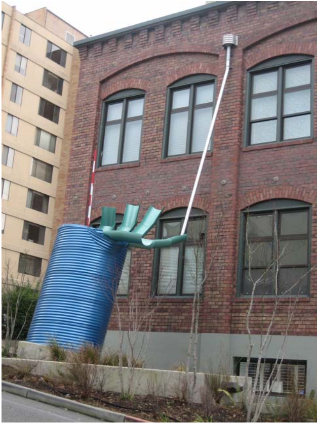
Figure 4 The sculptural “Beckoning Cistern” provides a durable rain message, reaching its hand to the building downspout to receive rain. A cistern valve opens to send rain into planters downhill. Design: Buster Simpson; photograph: Stuart Echols, 2013.
